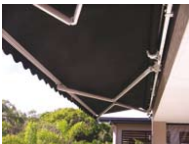
Amount of pitch available with the adjustable pitch control option
